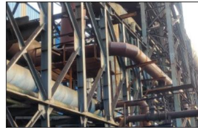
Dia- 600 mm pipe tapping from L.D. gas line (dia- 1400 mm)
